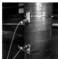
Installation of coated pipes
