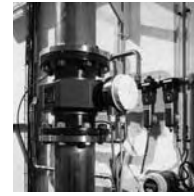
Flowmeters mounted in a fluid riser vertical pipe
