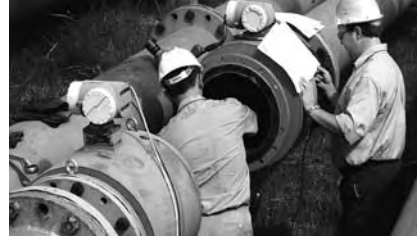
Inspection of the flowmeter pipe
