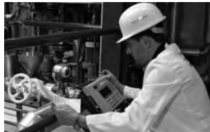
On-site calibration of pressure devices
